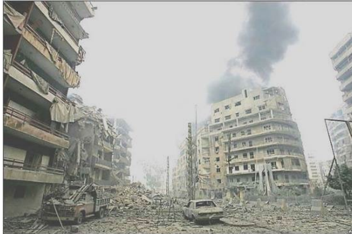
Figure 20: Example of MDZ-Like Blast Damage
